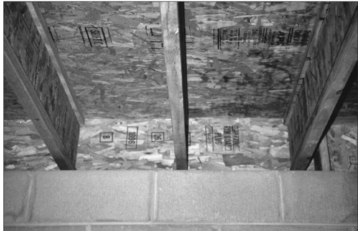
In this application, an engineered wood Rim Board is installed between the foundation sill plate and the floor under a wall section. The Rim Board matches the depth of the I-joists used in the floor framing.
